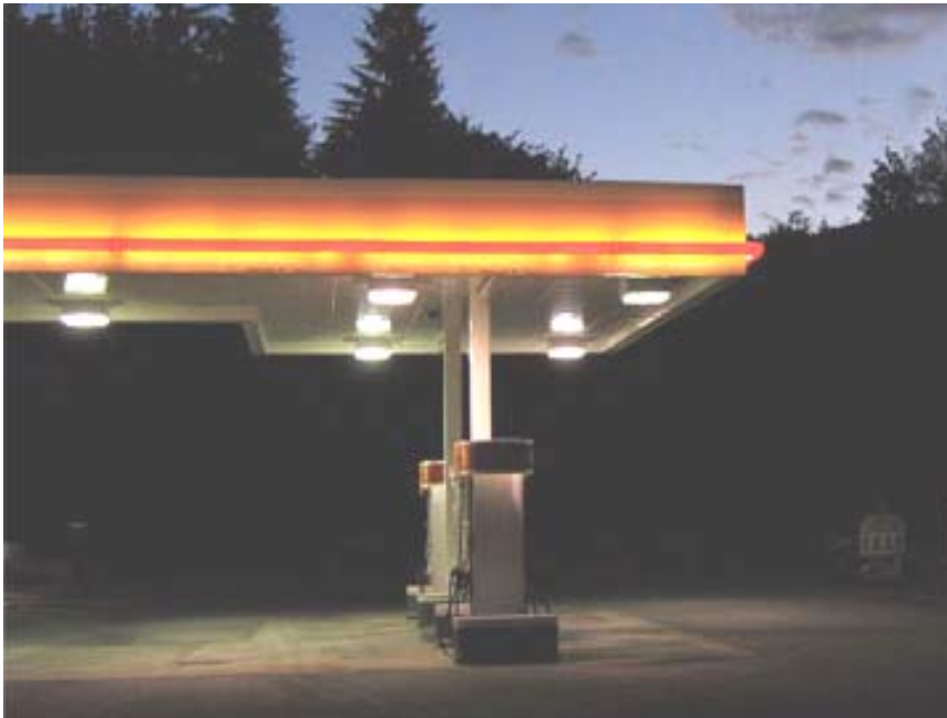
Example of drop lenses in a filling station canopy.
