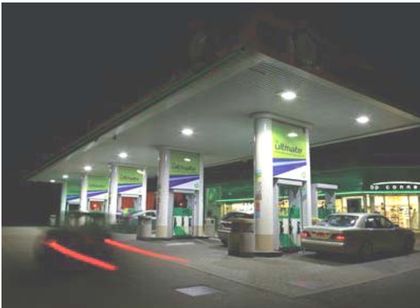
Example of flush lenses, which decrease glare and light pollution.
